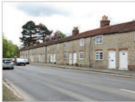
Simple Terraces with Arched Window Heads at Ground Level and Timber Lintels at Eaves
