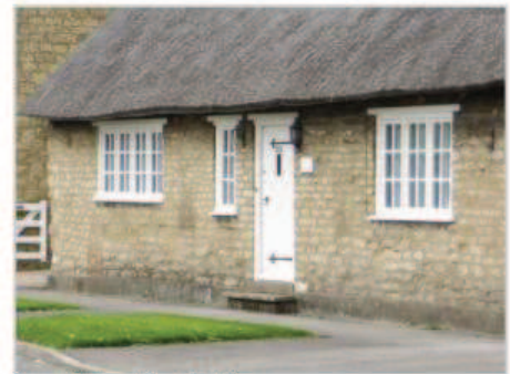
Casement Windows and Boarded Front Door
