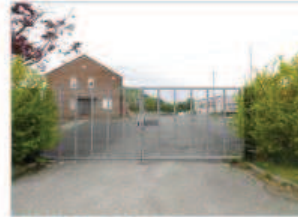
The Former Highway Depot
