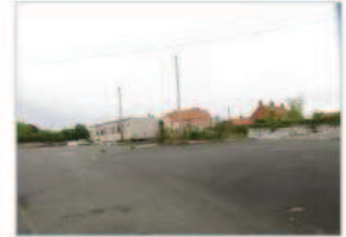
The Former Highway Depot
